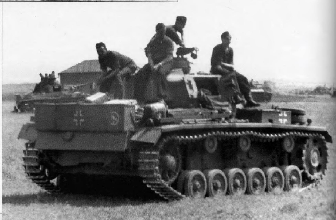
Another Pz.Kpfw.III Ausf.J from Pz.Rgt.24 of the 24.Panzer-Division. The large stowage box on the rear of the engine deck was a fitting peculiar to this division.
