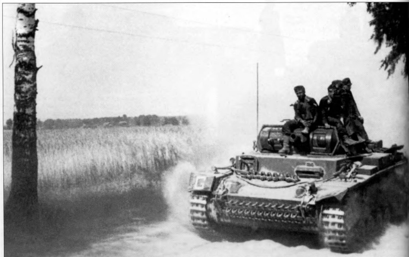
This early Pz.Kpfw.III Ausf.G converted to a Tauchpanzer is missing its 3.7cm gun barrel, leaving the armored barrel sleeve completely open. The white 'G' painted on its right fender indicates it belongs to one of the Panzer-Divisions assigned to Panzer-Gruppe 2 commanded by Generaloberst Heinz Guderian; in this case, 18.Panzer-Division. (Photo courtesy of John Prigent)
