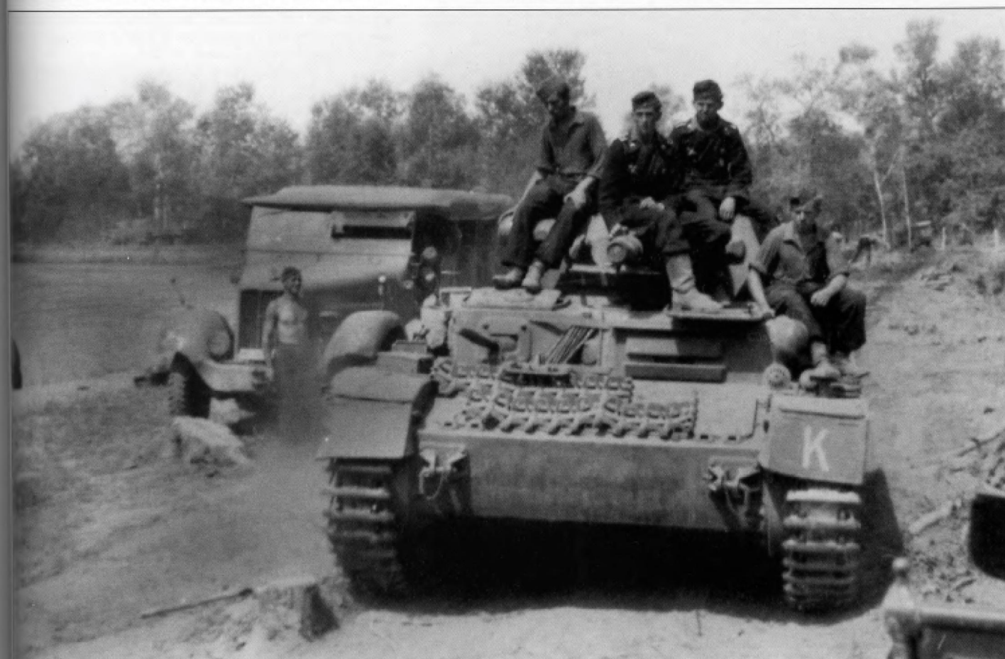
A Pz.Kpfw.IV Ausf.D from one of the Panzer Divisions assigned to Gruppe von Kleist during Operation 'Barbarossa' in June 1941. Whereas the Pz.Kpfw.IV Ausf.B and C were fitted with a straight front plate on the superstructure, the Pz.Kpfw.IV Ausf.D featured a stepped plate arrangement similar to the one on the Pz.Kpfw.IV Ausf.A. A white outline rhomboid with a '3' beside it can be faintly seen on the upper left side of the front plate.
