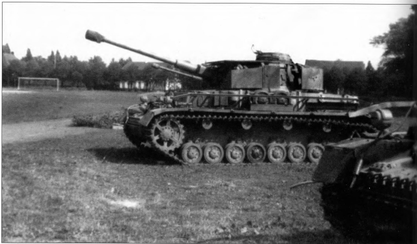
The steel angle that supported the hull Schürzen can be seen in this photo of a Pz.Kpfw.IV Ausf.G that has also been fitted with the 7.5cm KwK L/48 gun, also introduced in April 1943. The Schürzen plates themselves have been stacked on top of the turret, probably for rail transport. The camouflage paint scheme has been painted on the inside of the turret Schürzen access doors.
