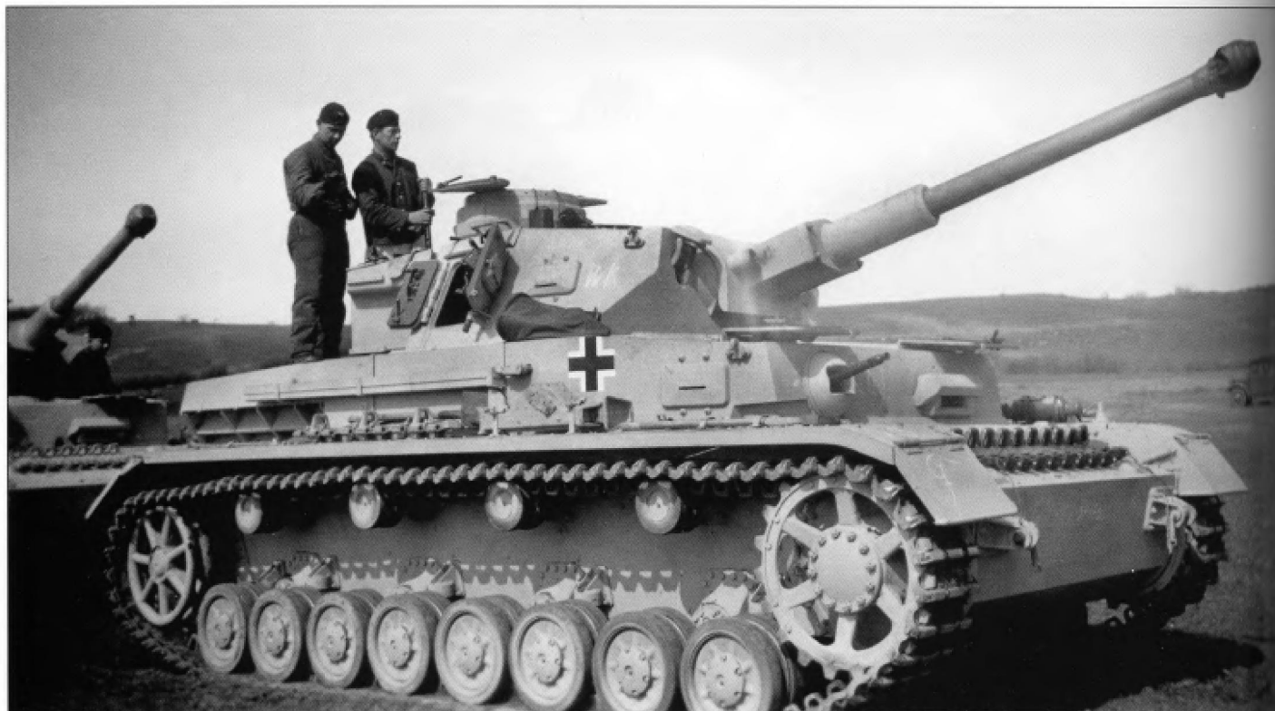
This new Pz.Kpfw.IV Ausf.F2, produced in March 1942, has been painted with a tropical color scheme of 2/3 Braun RAL 8020 and 1/3 Grau RAL 7027 for deployment to North Africa. The only external difference between the Ausf.F and Ausf.F2 was the new 7.5cm KwK L/43 gun. Initially, it was named Ausf.F2 but this was officially changed on 1 July 1942 to Ausf.G. The object lying on top of the hull beside the turret is the canvas dust cover for the hull machine gun.
