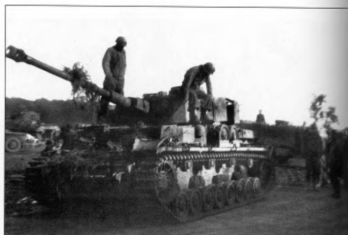
A group of American soldiers inspect what appears to be a relatively intact Pz.Kpfw.IV Ausf.J. The vehicle has a mixture of hub caps on the road wheels with at least one early style mounted on the front road wheel.
