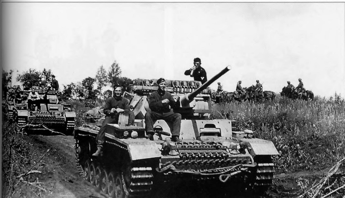
A column of Pz.Kpfw.III Ausf.J or L drive past mounted infantry from a Kavallerie regiment in Russia. The tactical emblem of 8.Panzer-Division, a 'Y' with a short vertical line beside it, can be seen painted in black on the front plate beside the driver's visor. The crew have wound a tow cable around the front of the vehicle using the 'S' tow hooks for quick use if needed.
