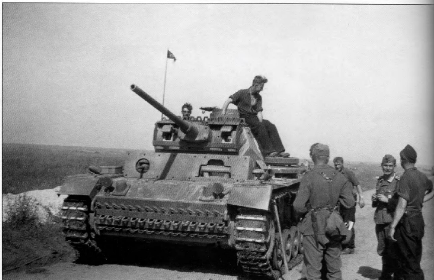
This Pz.Kpfw.III Ausf.J or L has been fitted with S-mine dischargers on the fenders, probably scavenged from a damaged Tiger I. Part of the tactical number '8' can be seen painted on the side of the turret.
