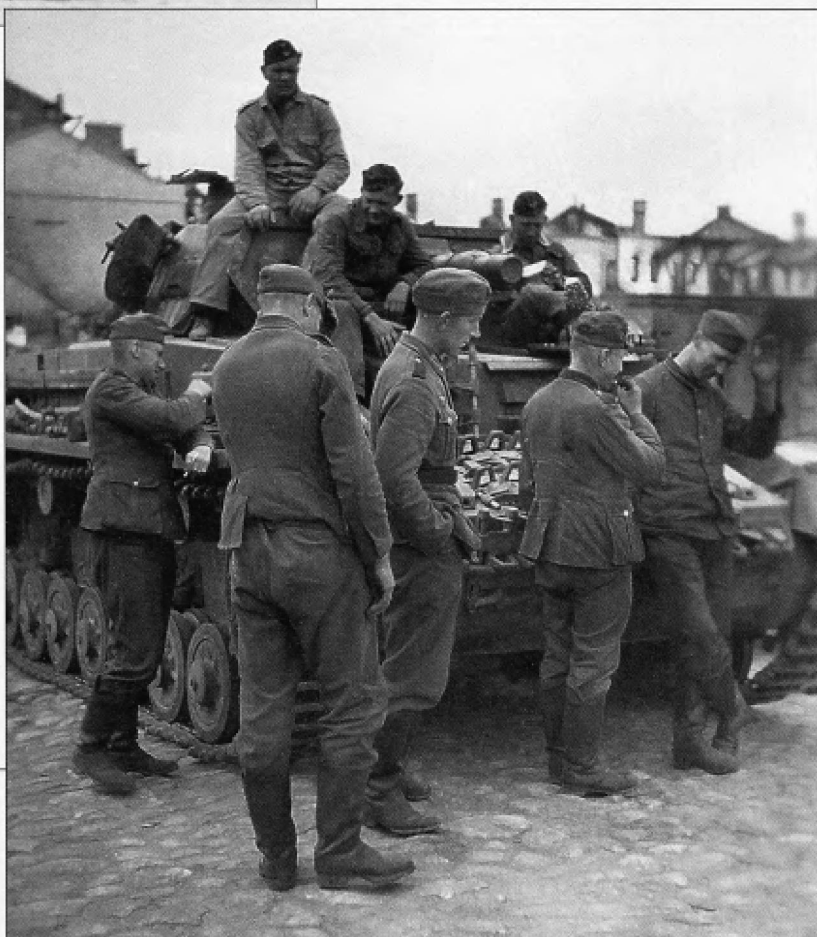
The crew of this Tauchpanzer IV Ausf.D and some infantrymen share a moment of camaraderie. The flange that the watertight mantlet cover was bolted to can be seen along the right side and top of the turret. A total of 48 Pz.Kpfw.IV Ausf.D were converted to Tauchpanzer in July and August 1940.
