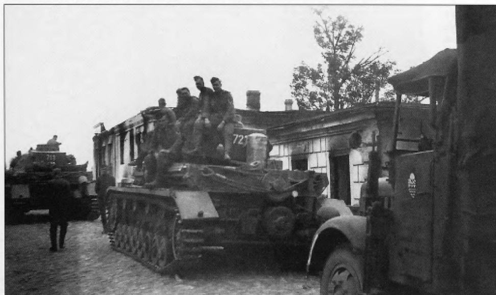
This Pz.Kpfw.IV Ausf.D has been fitted with additional 30mm armor plates to the front and sides of the superstructure and sides of the hull that were introduced in July 1940. The tactical number '51' is unusual in that Pz.Kpfw.IV's were normally assigned to either the 3. or 6.Kompanie in Abteilung with three companies or the 4. or 8.Kompanie in Abteilung with four companies.
