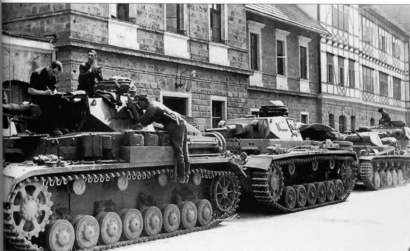
A Pz.Kpfw.IV Ausf.E converted to a Tauchpanzer from 8./Pz.Rgt.35 of the 4.Panzer-Division. A Pz.Kpfw.III Ausf.G can be seen behind it along with a Pz.Kpfw.II and another Pz.Kpfw.III converted to a Tauchpanzer. Additional 30mm armor plates were fitted to most Pz.Kpfw.IV Ausf.E and can be seen on the front and sides of the superstructure and sides of the lower hull.
