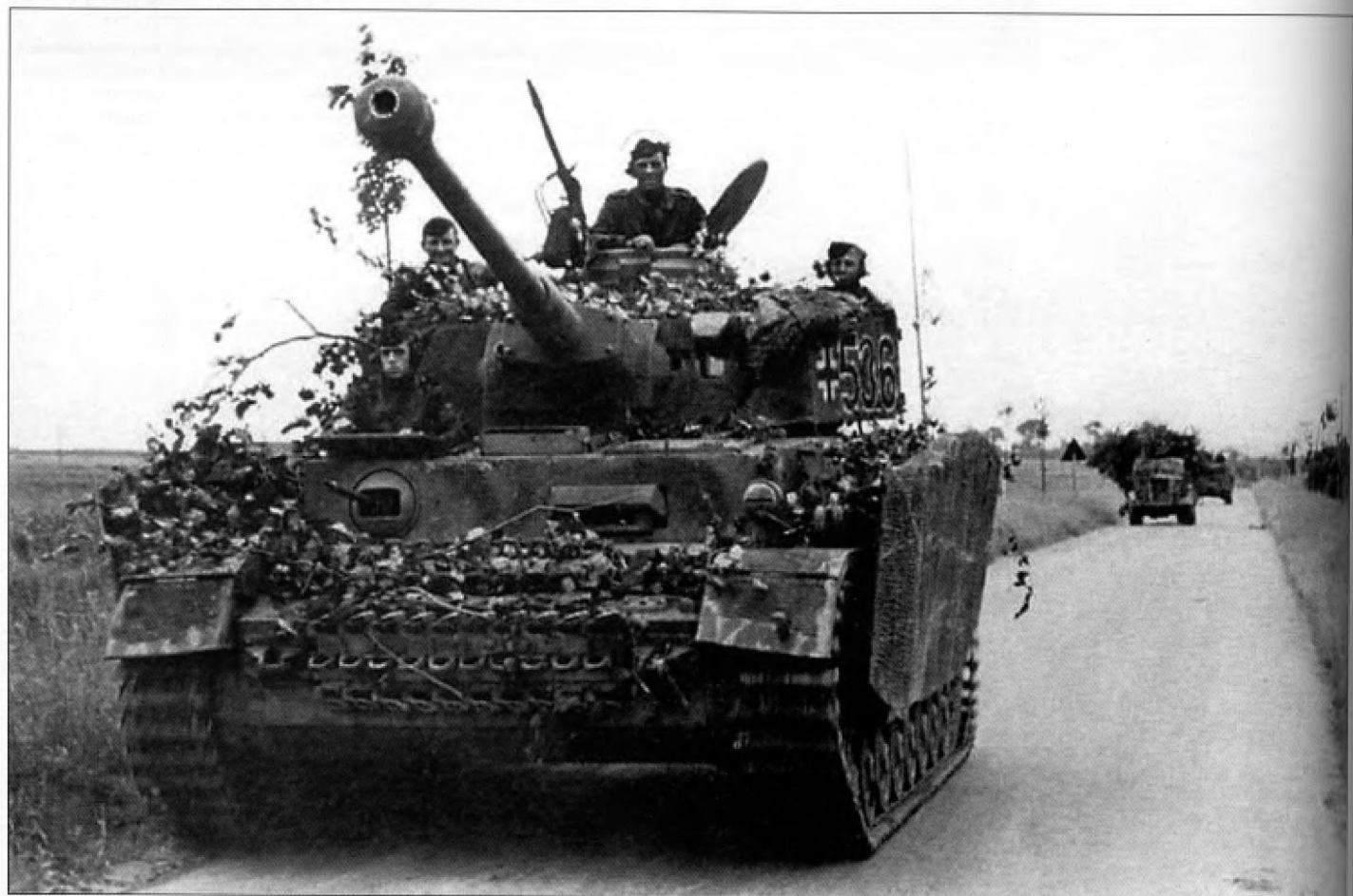
Beginning in September 1943, Zimmerit anti-magnetic mine paste began to be applied to the Pz.Kpfw.IV Ausf.H including this one from 5./SS-Pz.Rgt.12 from the 12.SS-Panzer-Division seen here in Normandy. Initially, Zimmerit was applied to the hull as well as the turret and hull Schürzen plates but was soon applied only to the vehicle itself.
