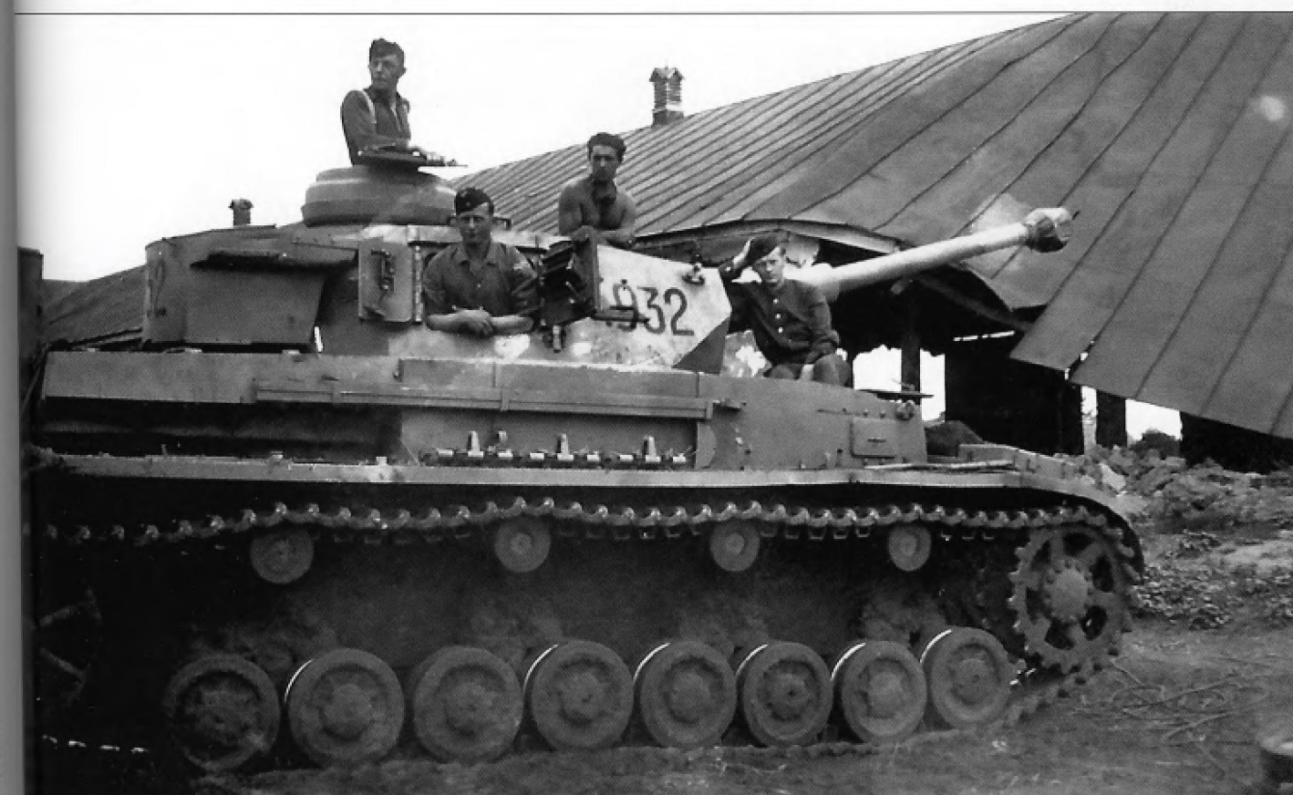
This Pz.Kpfw.IV Ausf.F2 is still fitted with the turret side visor indicating it was produced in March or April 1942. The outward appearance of the Pz.Kpfw.IV could not change significantly through to the end of the war.
