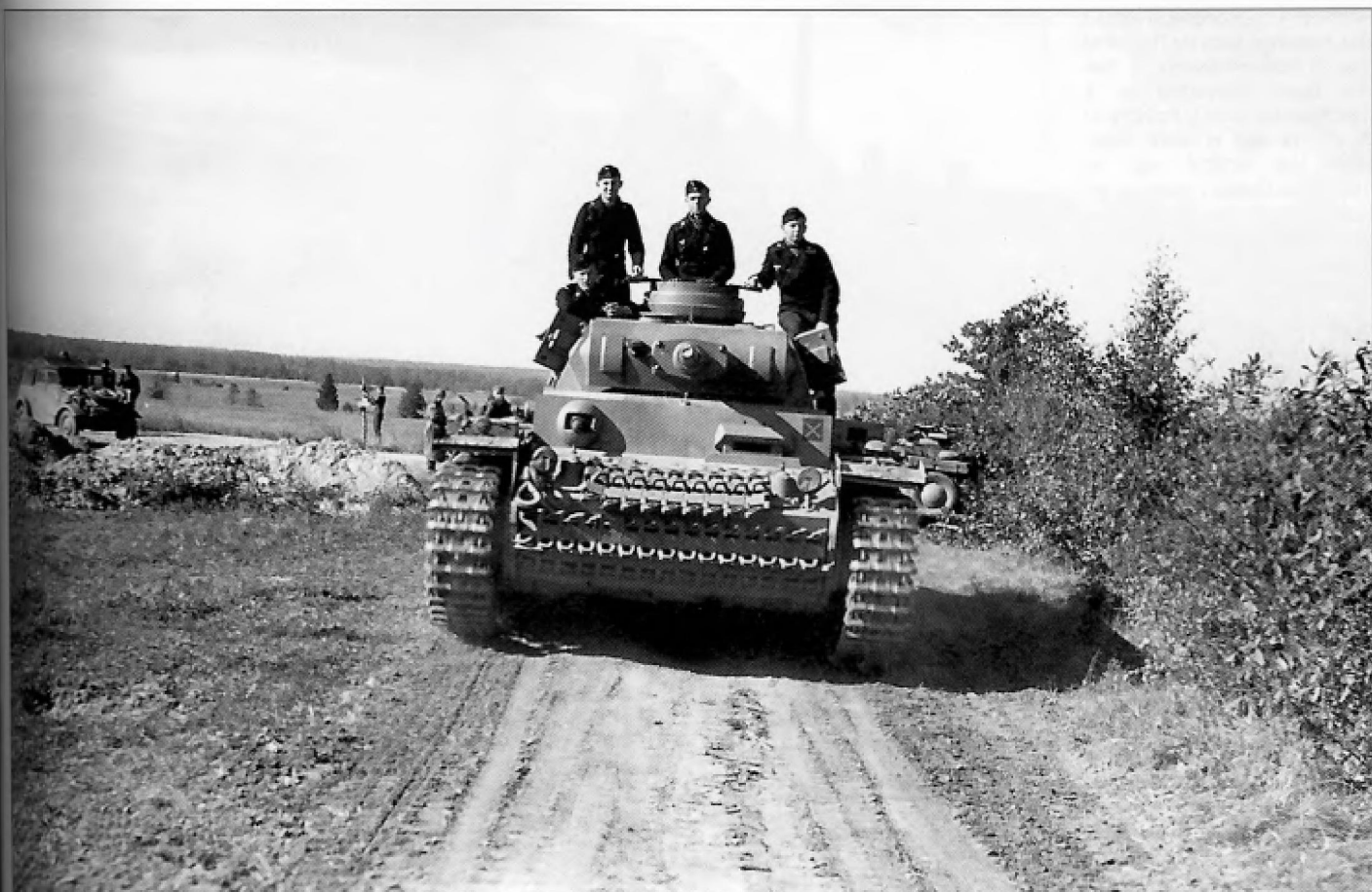
A Pz.Kpfw.III Ausf.J from Pz.Rgt.31 of the 5.Panzer-Division rolls down a dirt track in Russia in the summer of 1942. Track links carried on the front of the vehicle provided a small measure of extra armor protection in addition to their primary purpose of simply being spare tracks.
