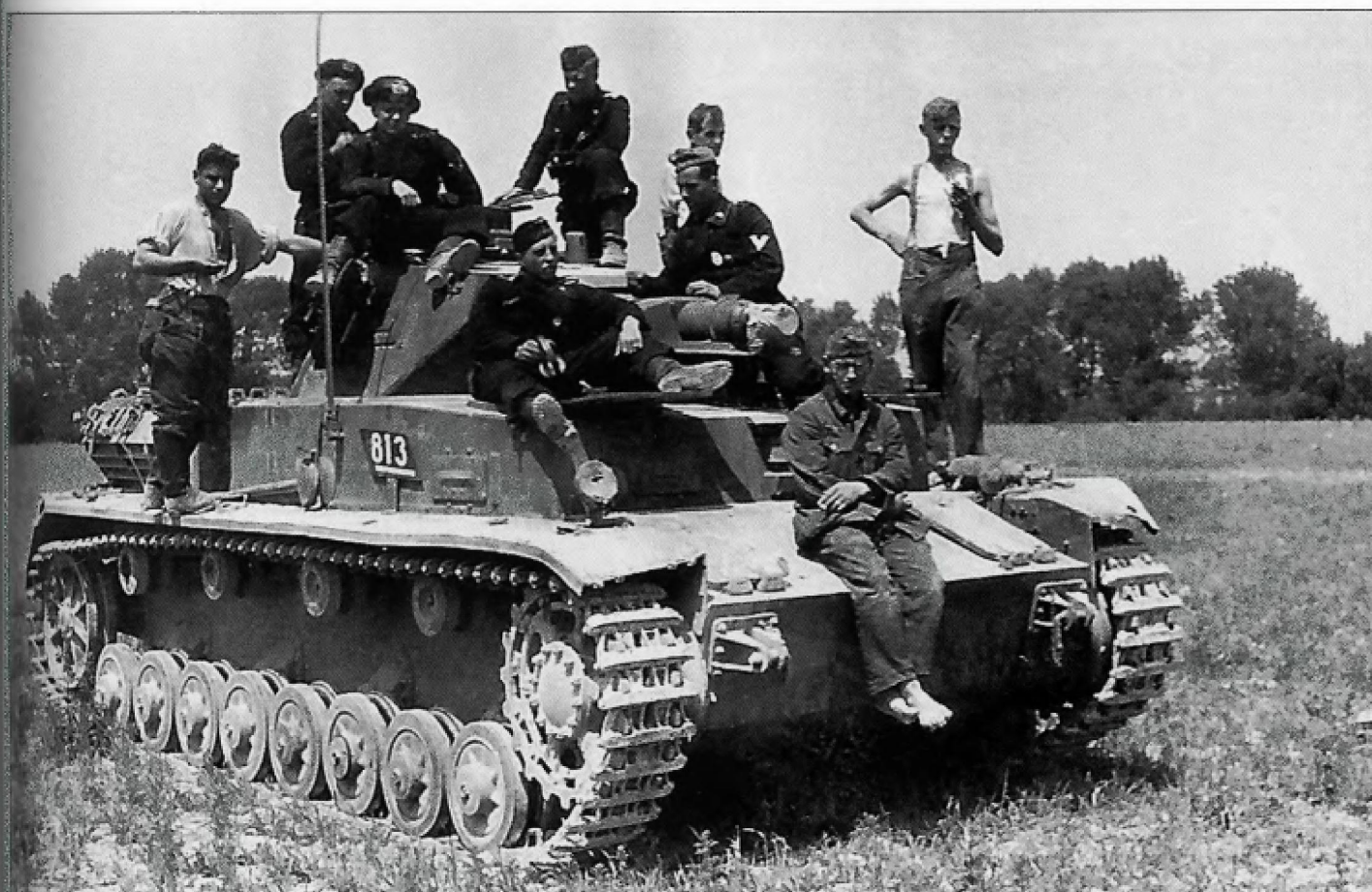
The wooden antenna trough is missing off this battle scarred Pz.Kpfw.IV Ausf.B or C along with most of the tools normally carried and the hinged mudguards. The tactical number '813' is painted in white on a black metal rhomboid plate following standard early practice. This would have been carried on both sides and the rear of the vehicle. Note how the dust has completely covered lower parts of the hull and running gear.
