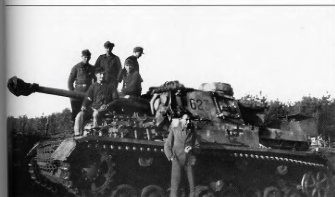
A Pz.Kpfw.IV Ausf.F and a Pz.Kpfw.IV Ausf.F2 from Pz.Abt. 'Großdeutschland' photographed on the Eastern Front during the summer of 1942. This photo provides a good comparison of the difference between the short and long barrel Pz.Kpfw.IV.
