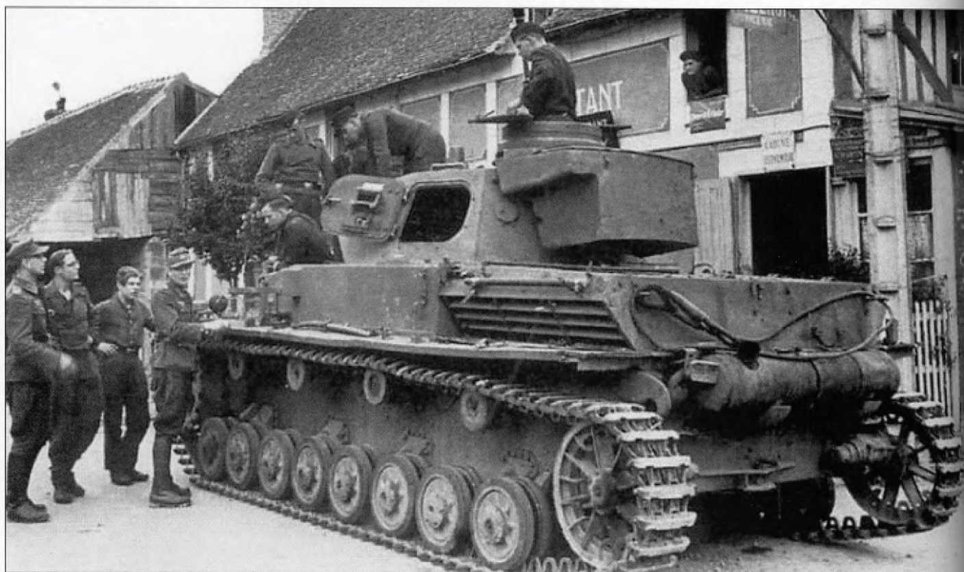
This Pz.Kpfw.IV Ausf.B soldiered on into 1944 where it is seen here with Pz.Rgt.22 of the reformed 21.Panzer-Division in France just before D-Day. The division was poorly equipped and had 21 obsolete Pz.Kpfw.IV with the 7.5cm KwK L/24 in its inventory at this time. Missing most of its tools and equipment, it doesn't look ready for combat.
