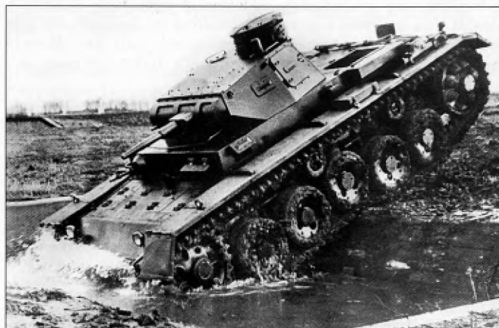
A Pz.Kpfw.III Ausf.A negotiates a water filled ditch during a training exercise during the pre-War years. The five large road wheels utilized a coil spring suspension and the maximum armor thickness was 15mm. Only ten vehicles were produced in 1937, seeing action in Poland in 1939 before being withdrawn from service in early 1940.
